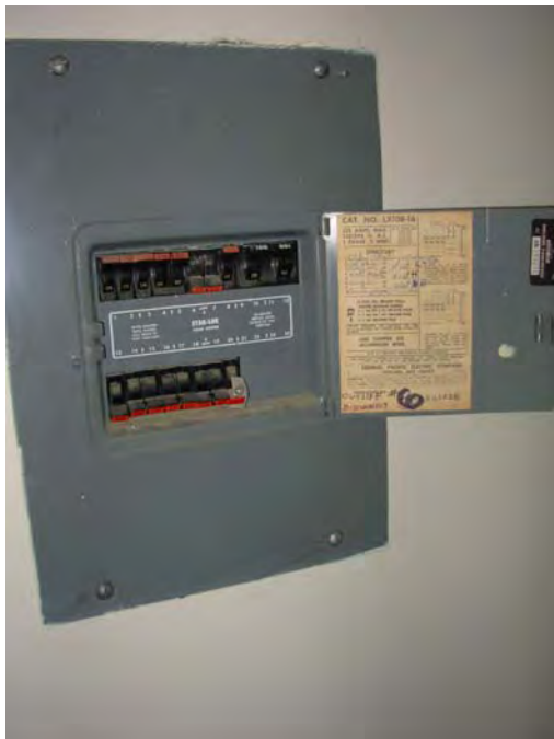
15. FPE Stablok circuit breaker panels to replace Murphy Apartments • Capital Needs Assessment • © On-Site Insight
