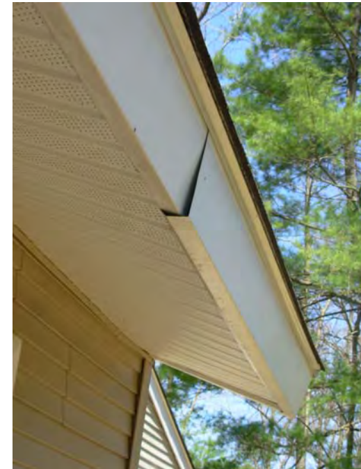
8. Spot seam separation at soffits
