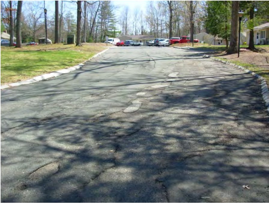
1. Patched asphalt paving at access roadway
