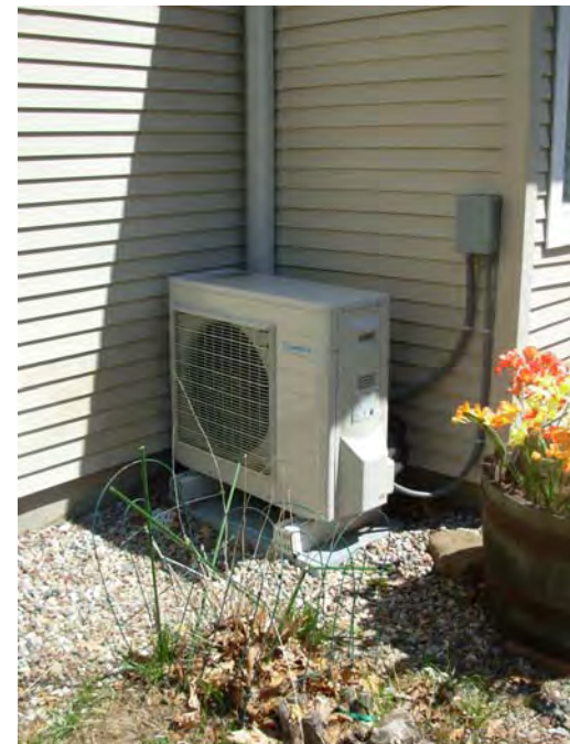
16. Heat pump HVAC system exterior condensers
