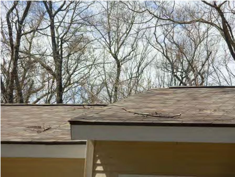
9. Roof decking deflection, note tree limbs
