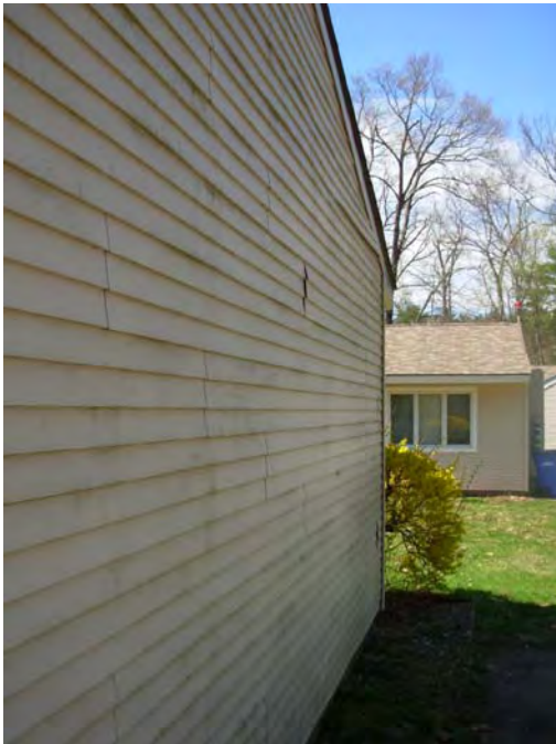
7. Spot damage and organic material growth on siding
